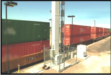
Radiation Monitoring System
