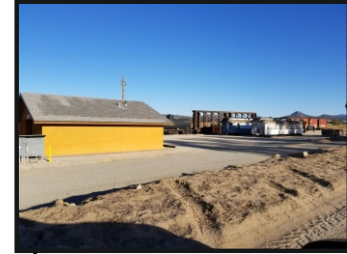
Pacific Southwest Railroad Museum (existing restrooms to be remain)
